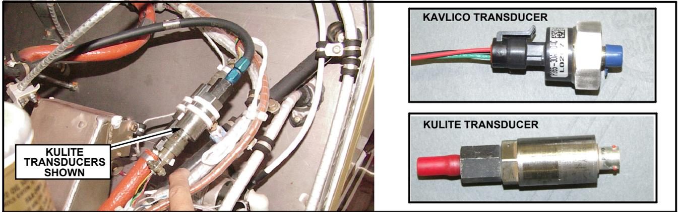
Figure SB M20-307-1 - TRANSDUCER IDENTIFICATION
